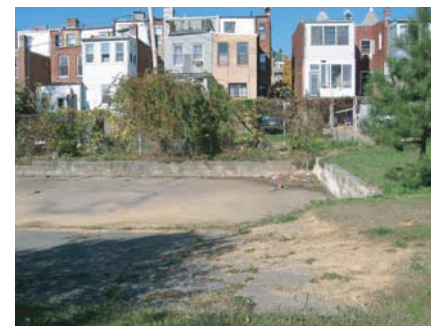
wall at pad
